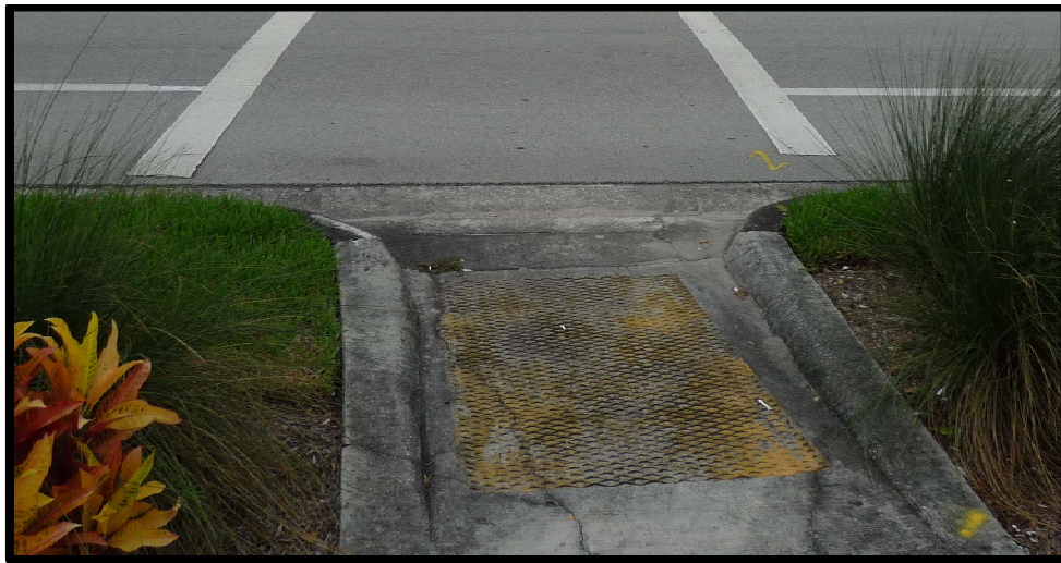
Figure 4: North-South Crosswalk Ramp in the Northwest Corner at Sunrise Drive
